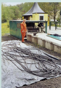
Left and above: Replacement of the cable at Vogtland-balloon
