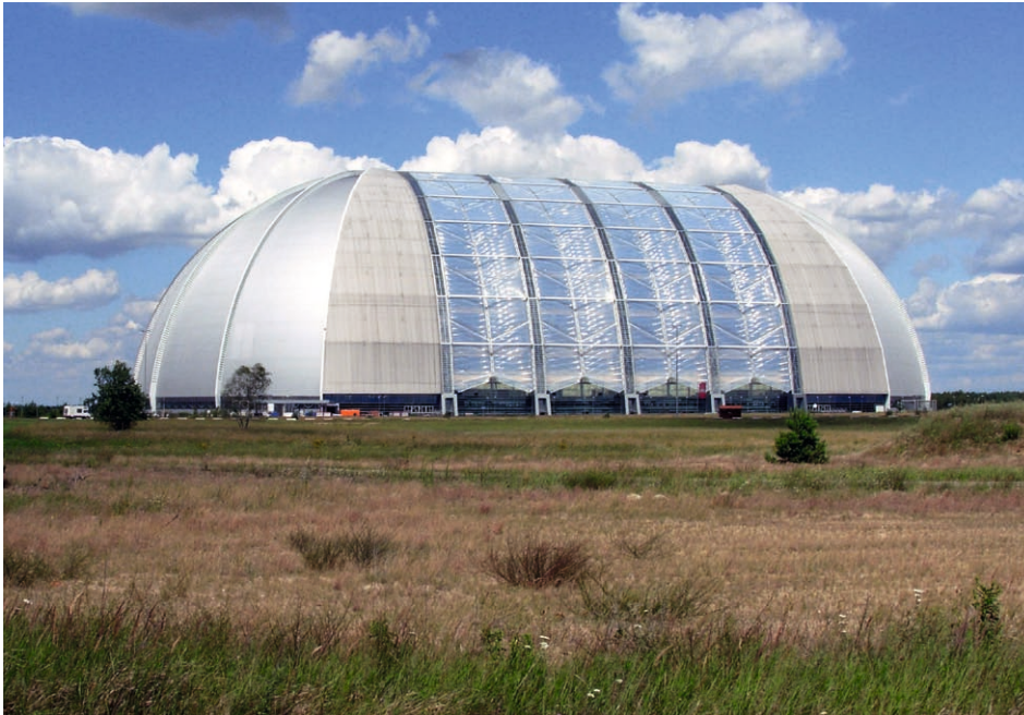
View aback: CargoLifter hangar, now Tropical Islands
